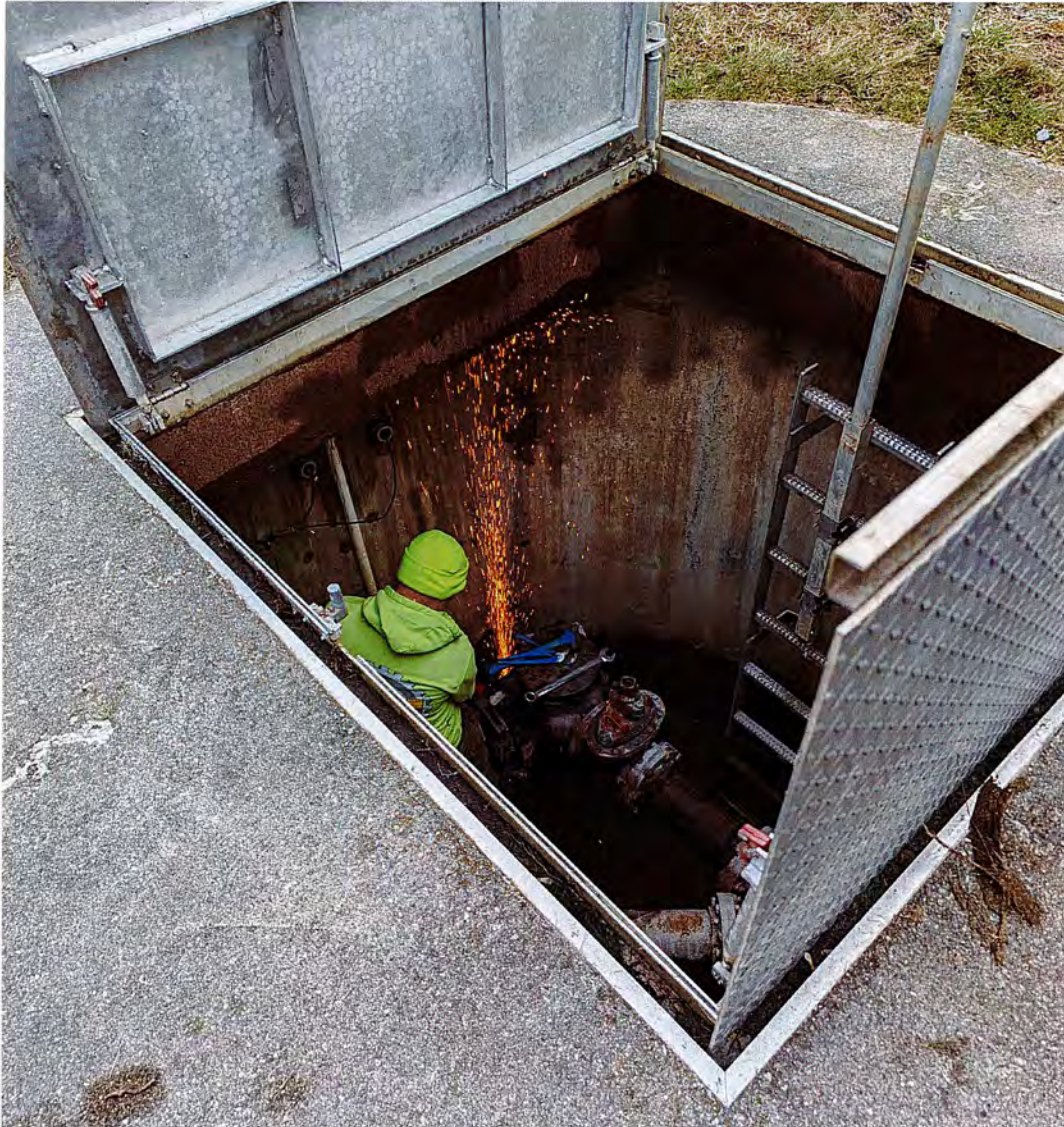
Check Valve Removal at Pump Station 71
