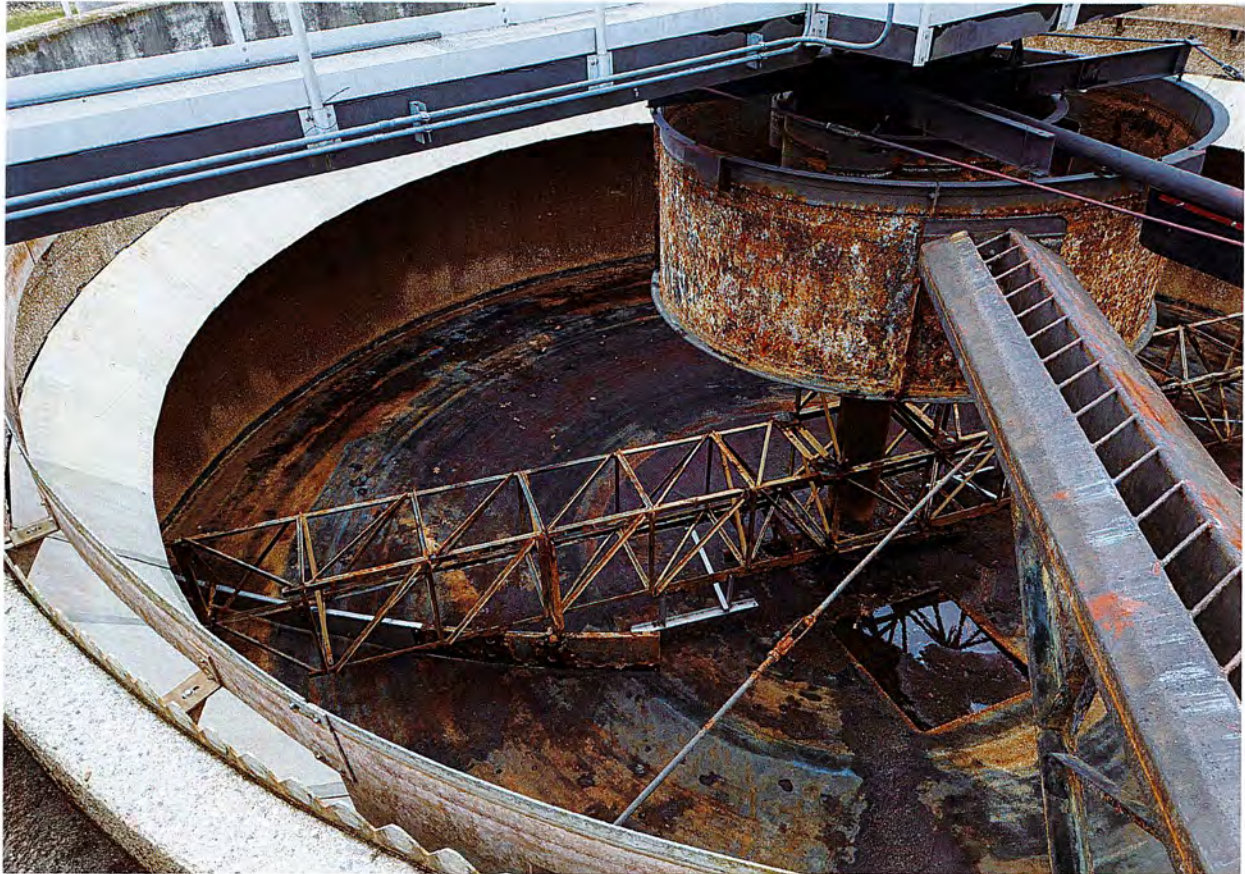
South Clarifier Repairs - New Fabricated Steel and Repaired Baffles
