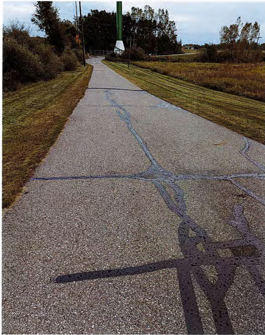
Crack Sealing and Patching of Driveway
