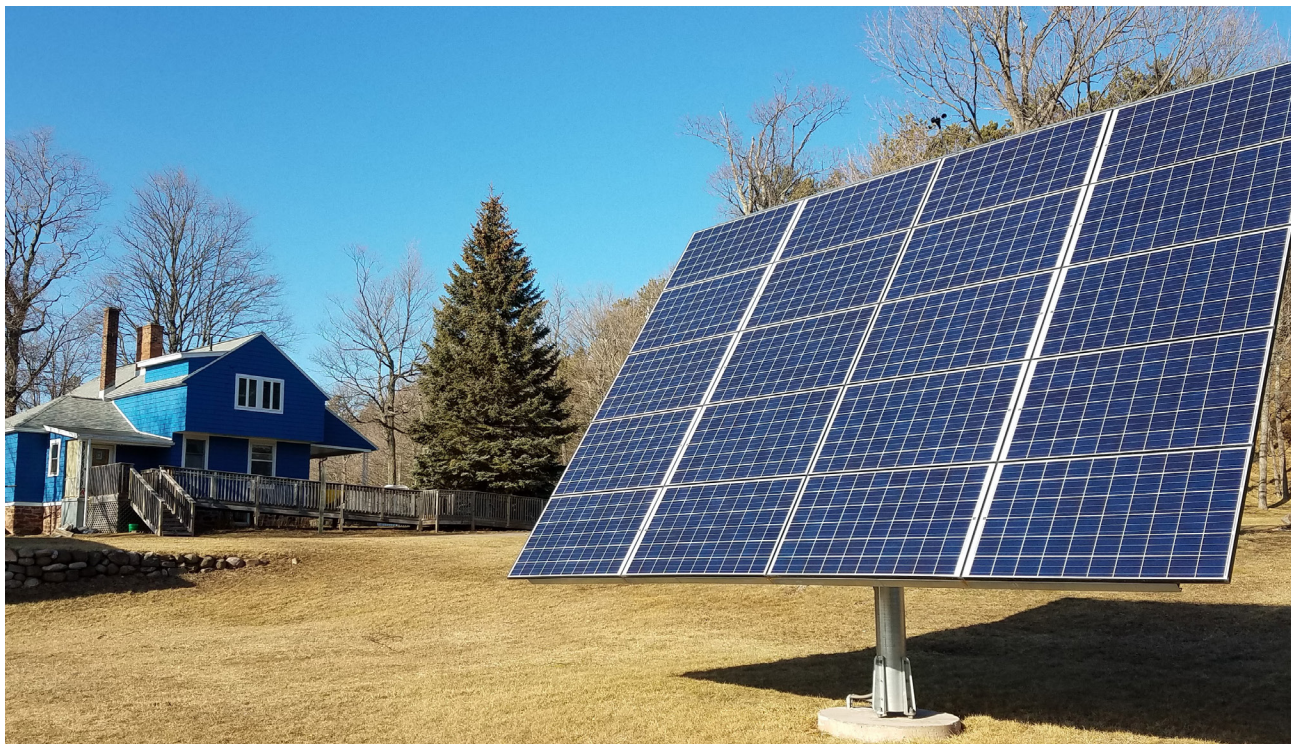
Ground-mounted monopole SES. Photo by Bradley Neumann.
