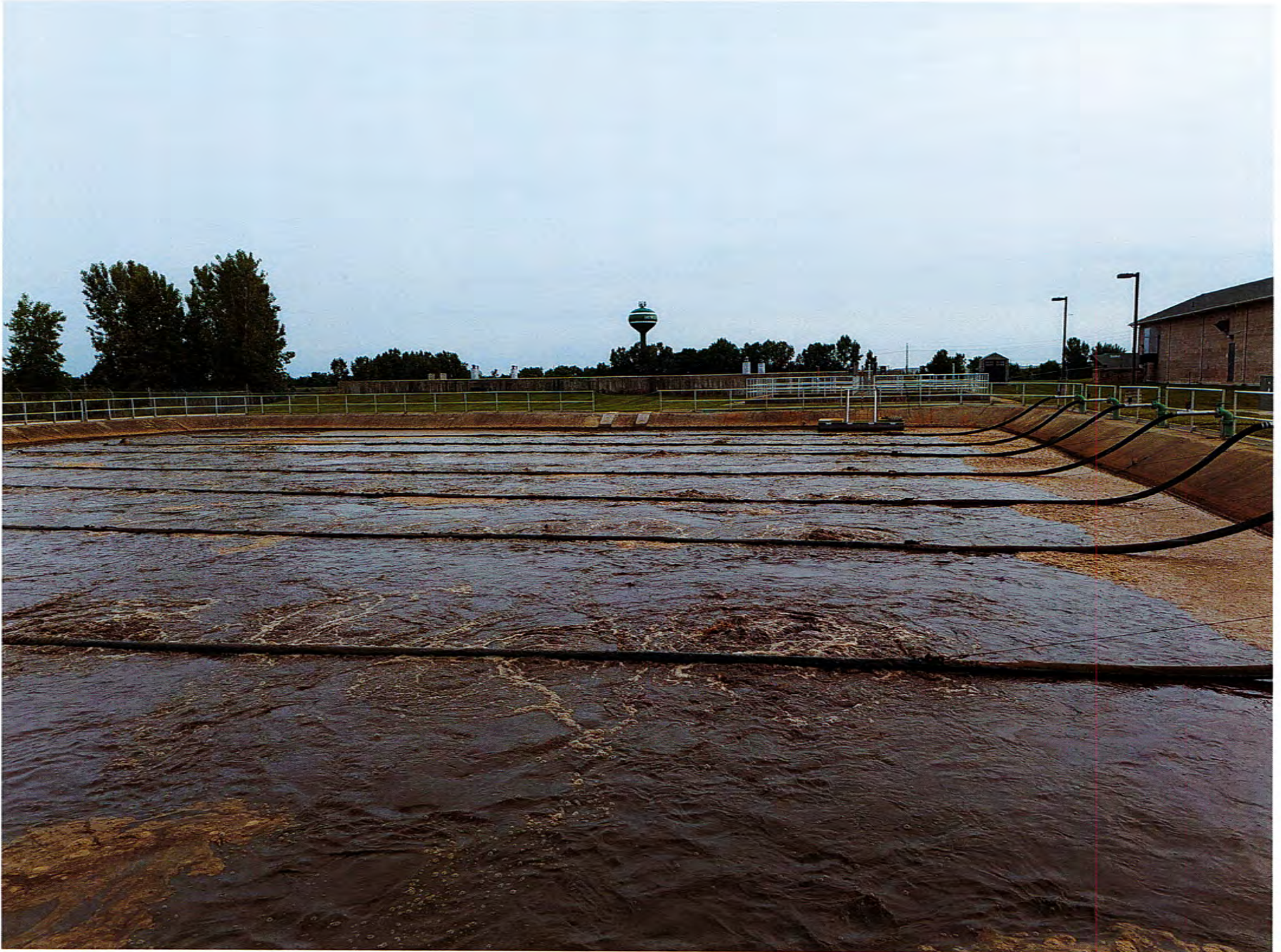
Bio-Lac Basin with All Aerators Repaired and Lower Air Input
