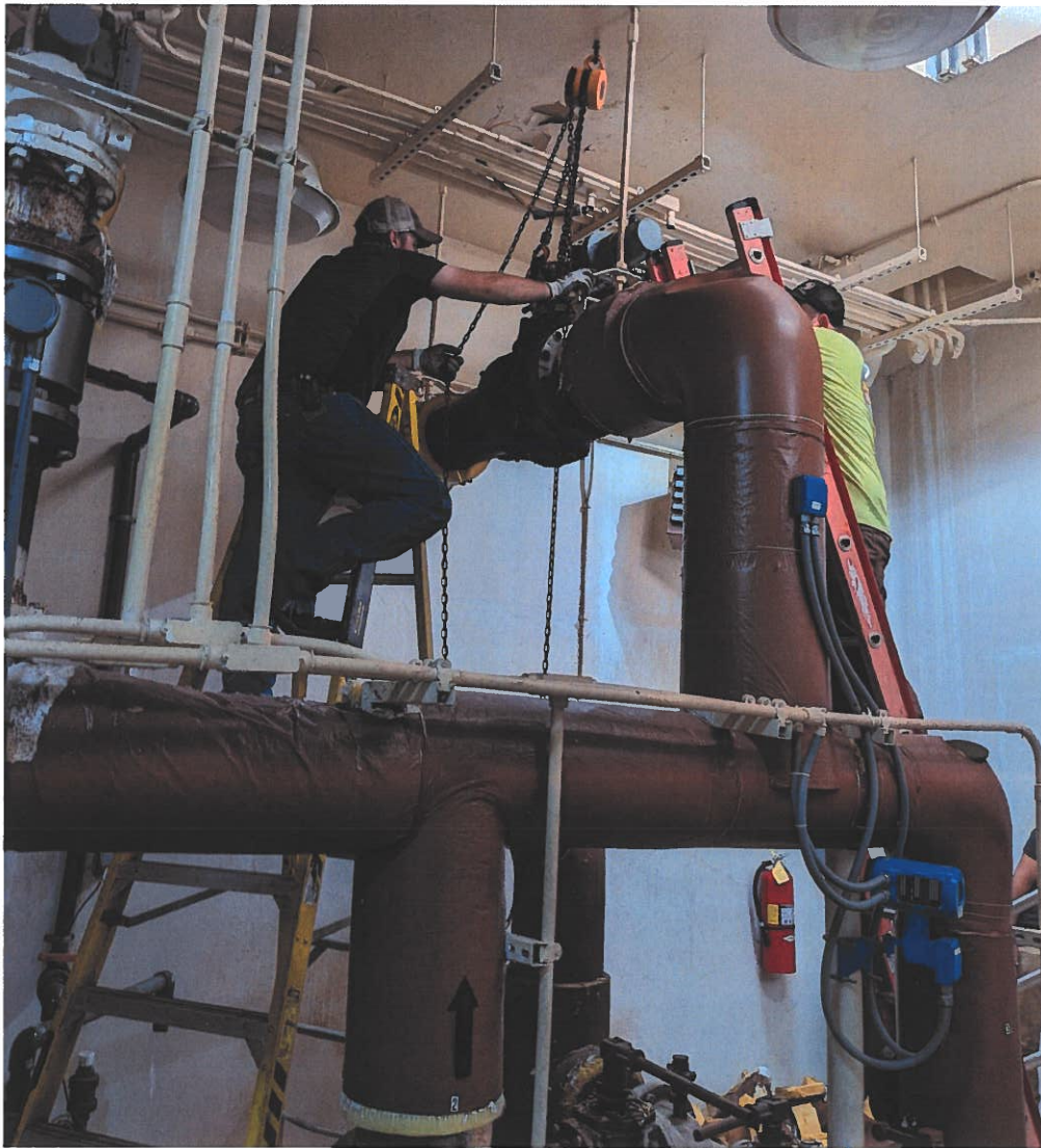
New Waste Valve and Actuator Installation
